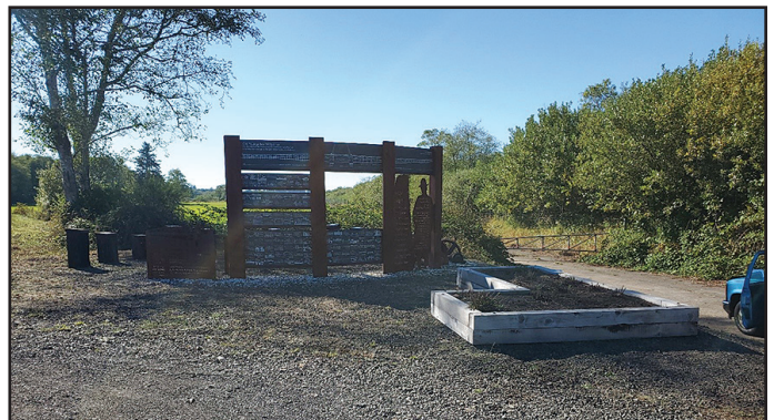
Clean-up Completed! Lewis & Clark River Bridge Wayside.
