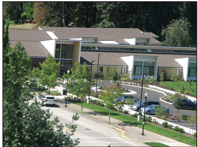
The completed project.
