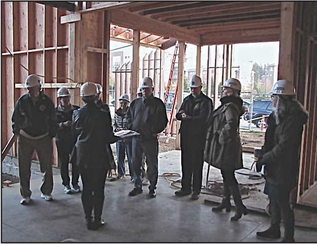
Lions tour as Heartfelt House is under construction.
