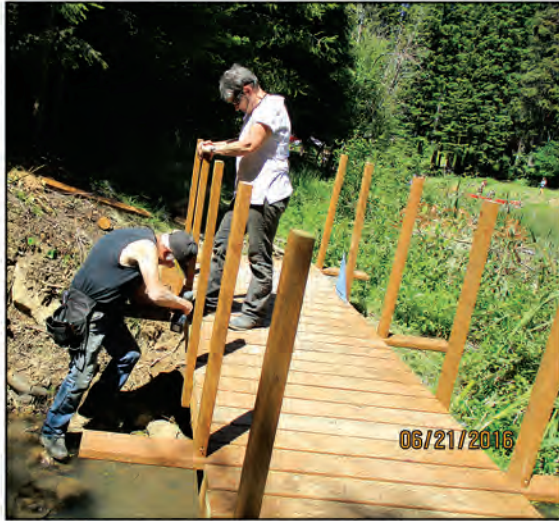
Lions Tony and DG Debi Castor working on the bridge
