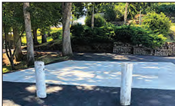
The new ADA parking spaces.
